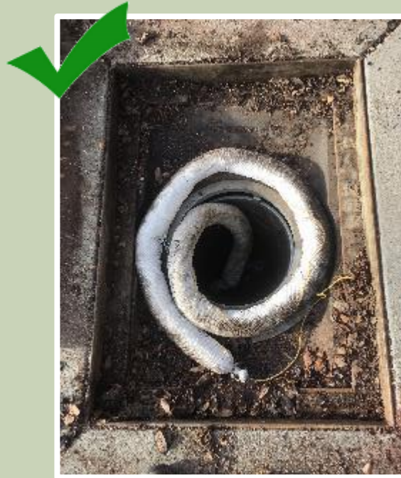
Filter fairly clean, oil absorbent still has capacity
