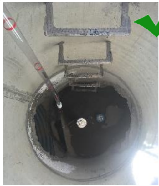
Use a “sludge judge” or similar to check for sediment in a separator’s sump
