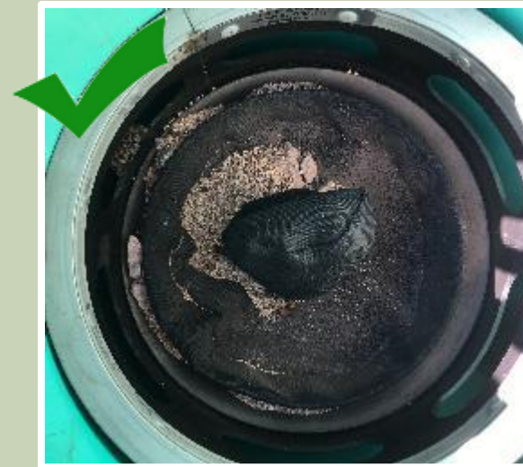
Filter has plenty of capacity
