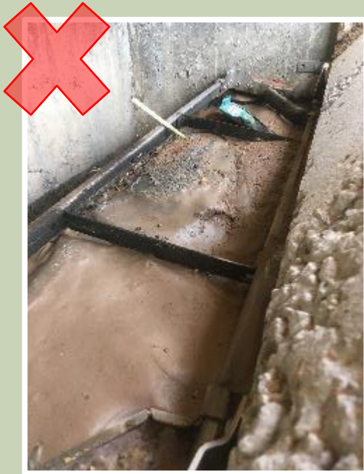
Filter completely full of sediment
