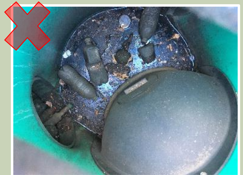
Nasty! Excessive oil indicates an illicit discharge occurred
