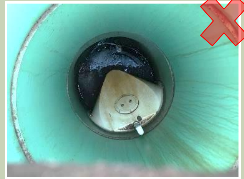
Sump is completely full of sediment & requires immediate maintenance
