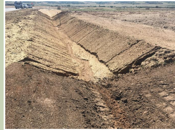
This ditch needs erosion control
