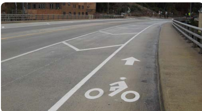
Buffered bicycle lane www.pedbikeimages.org /Lyubov Zuyeva
