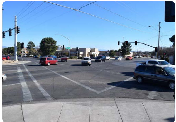
Above is the intersection of SR 89A and Main St., which currently lacks bicycle facilities.
