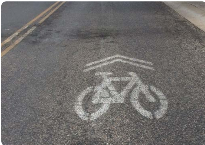
Regular maintenance includes repainting bicycle lanes and shared lane markings (“sharrows”).
